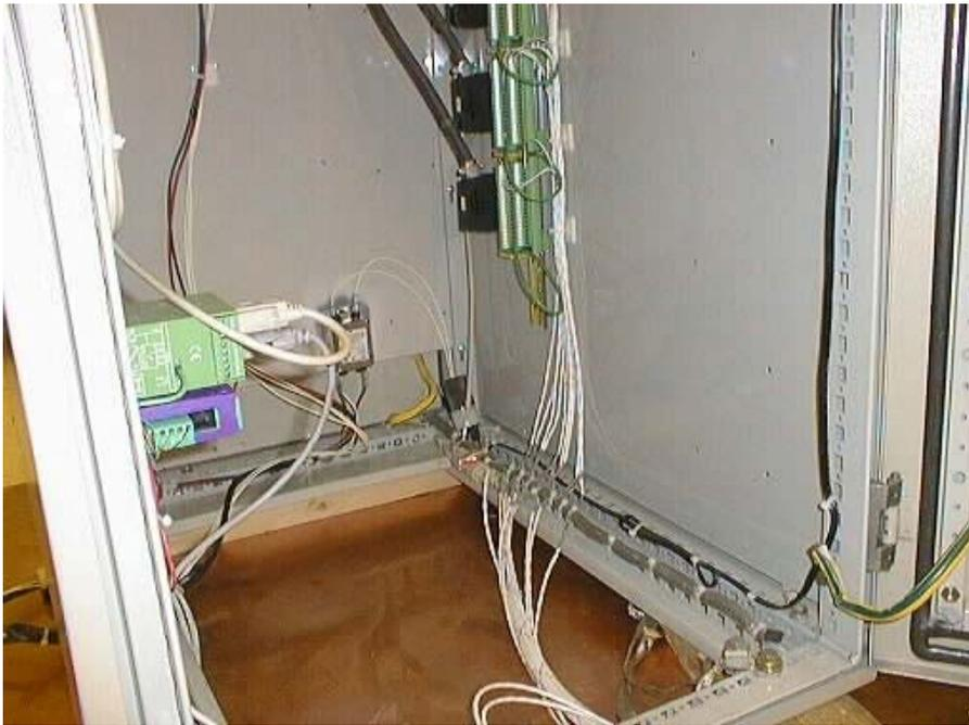
Figure 9-5—Bottom Cable Entry Area
